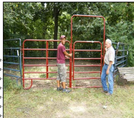
Karl Glueck & Lawrence Simms work to install the round panel gate donated by Karl & Velda Glueck.
